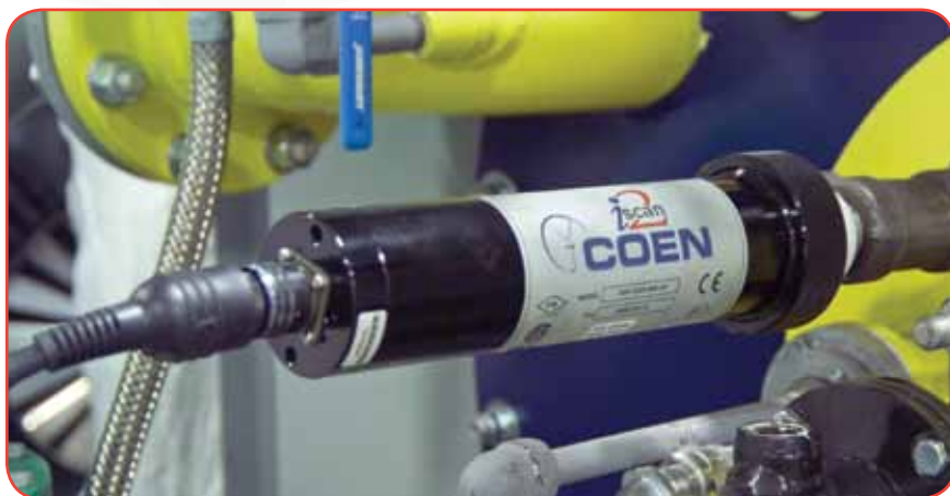
iScan2™ Flame Scanner for Enhanced Flame Detection, Self-Checking, HART COMMUNICATION PROTOCOL
